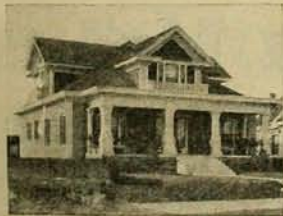
A No. 1-22-W IDEAL Boiler and 422 ft. of 3/8-in. AMERICAN Radiators, costing the owner $195, were used to Hot-Water heat this cottage.
